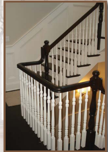
Two tone stairs with 4300 newels, 5300 paint grade balusters
