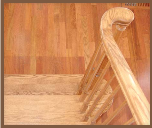
5015 Balusters 4010 PT Newel 6010 Top Rail LH Turnout
